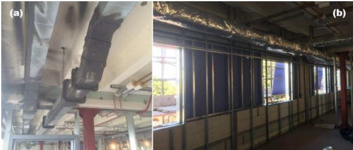
Figure D-9. Ductwork joint seals (a) alone that did not meet DALT criteria; insulation provided (b).
