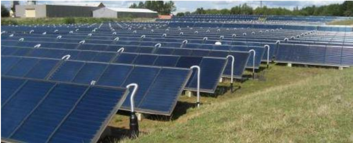
Figure C-9. Solar collector of 500 m 2 .
