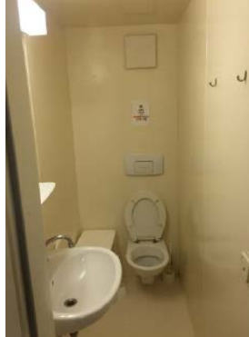
Figure A-5. Existing ventilation system exhaust air uptake in the sanitary rooms above WC.
