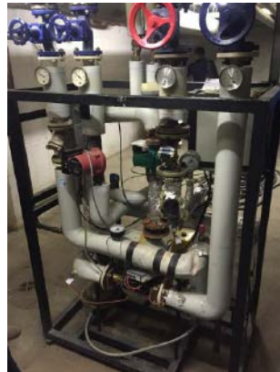
Figure A-6. Existing district heating station.
