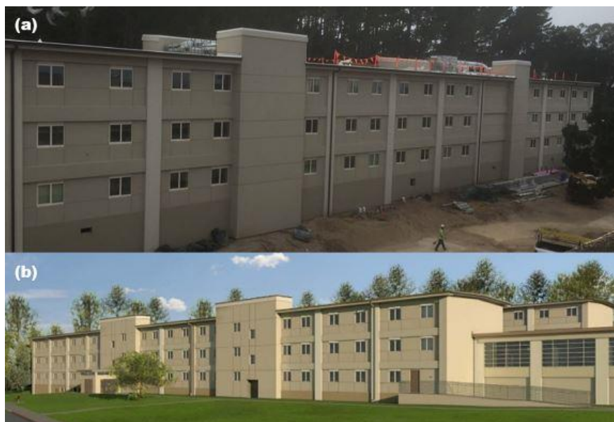
Figure D-12. Completed first wing of Presidio Bldg. 630.
