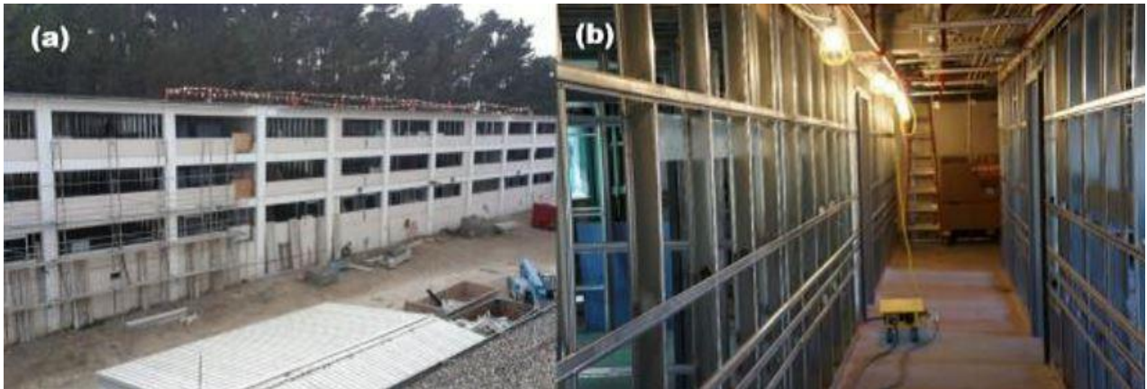
Figure D-6. Guttied exterior (a) and the interior (b) of Bldg. 630.
