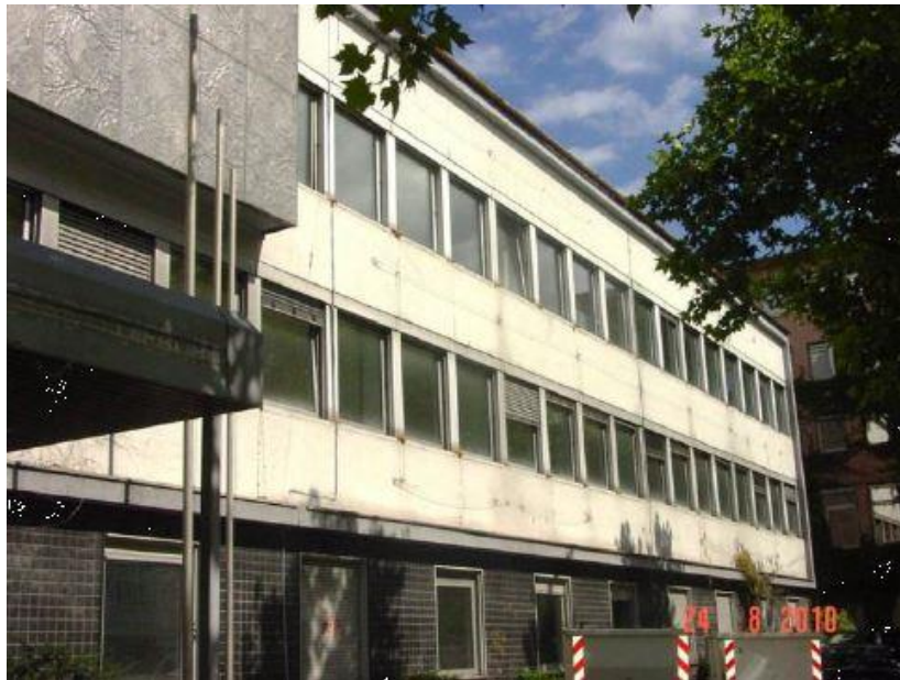
Figure B-1. Front view from the street on the southern part of the building before refurbishment (Darmstadt case study).
